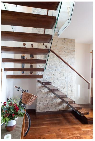
**PROJECT:** Timber clad steel staircase
